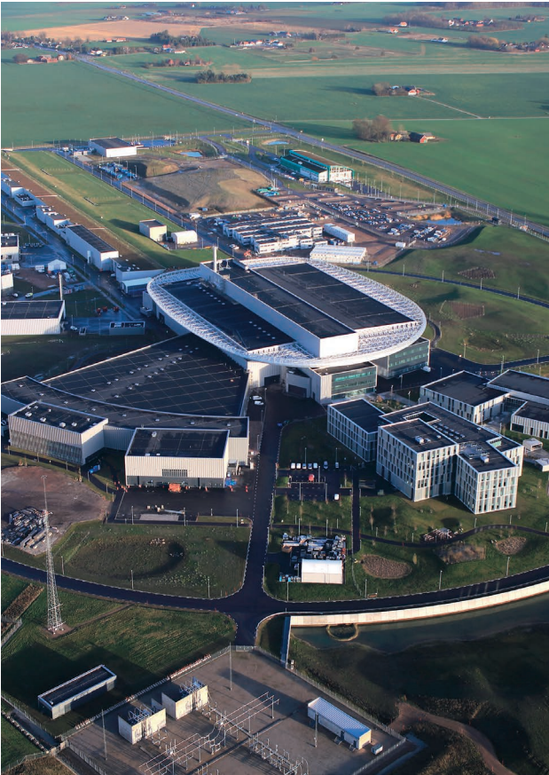
Aerial view of the ESS construction site in Lund, Sweden. Photo: ESS
