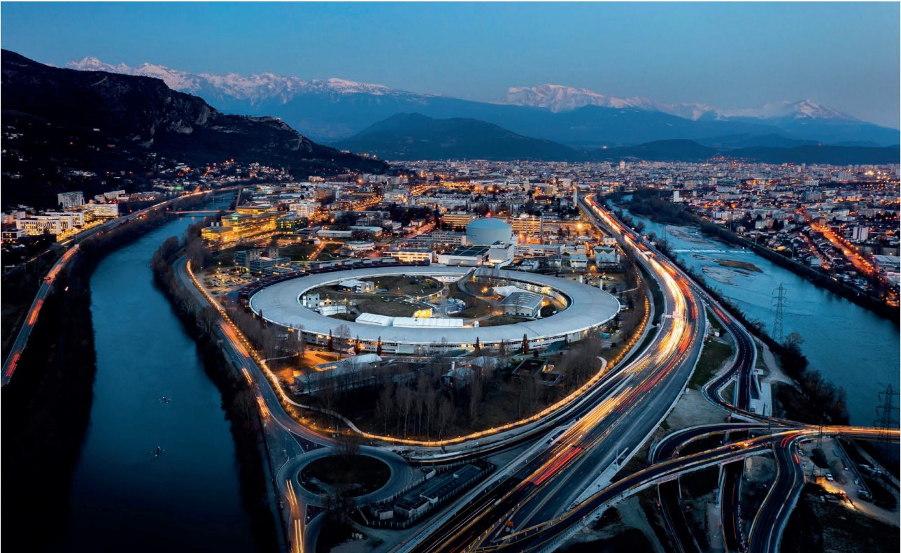
X-rays with exceptional properties are produced at ESRF by very high energy electrons circulating in a storage ring, a circular tunnel with a circumference of 844 m. Photo: ESRF/VUEDICI
